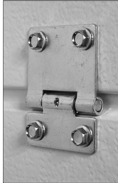
Figure 30: FS intermediate hinge installed
